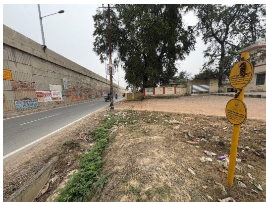
Photo 6: Gas Grid Connection Point
